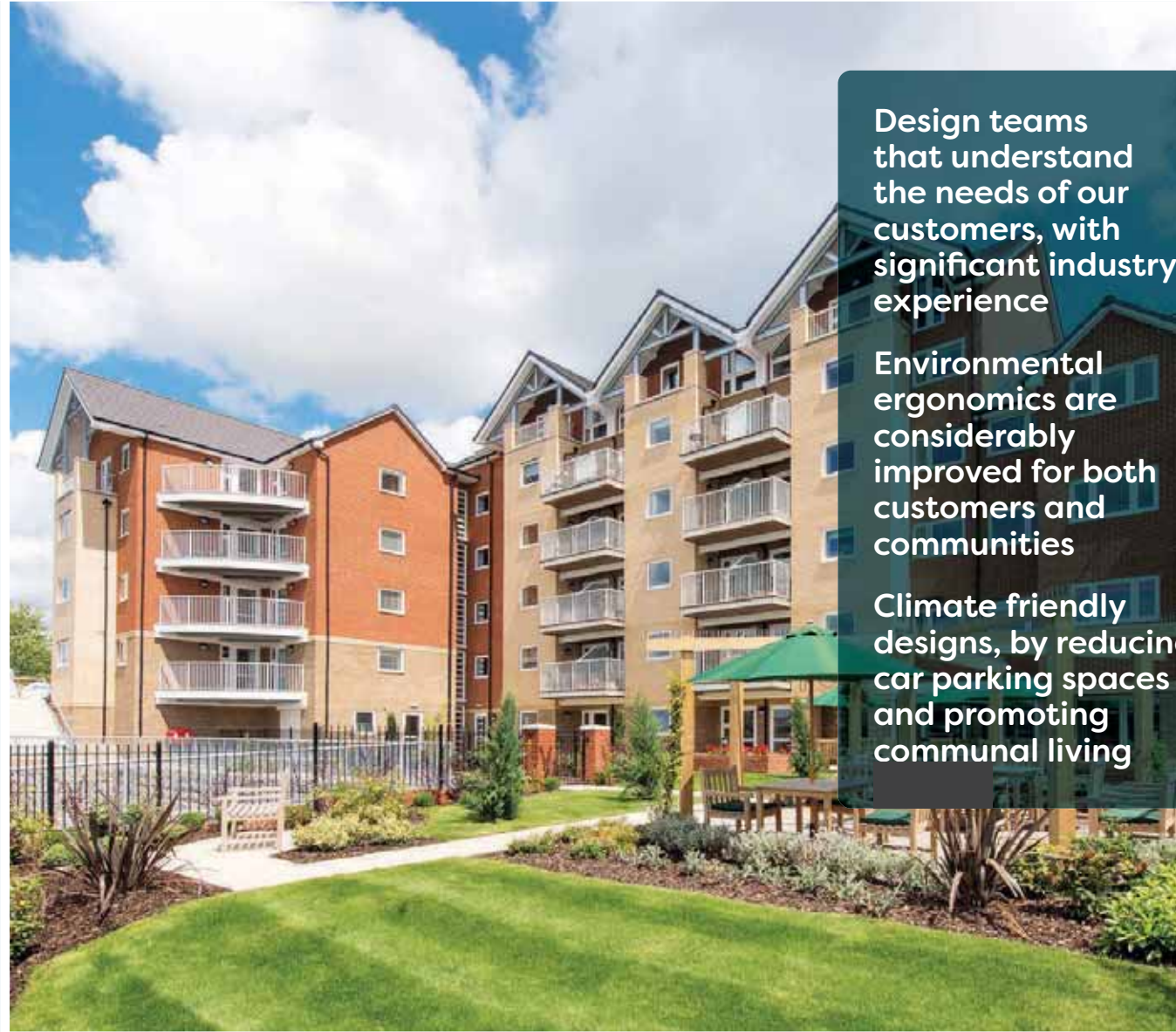
The Boathouse, Southampton, Hampshire
